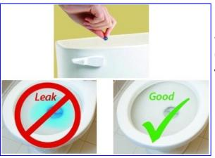
• Check your toilets for leaks. (Put food coloring in your toilet tank. If, without flushing, the color begins to appear in the bowl, you have a leak that should be repaired.)
