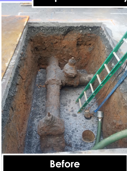
Chestnut Street Valve Replacement & Hydrant Installation
