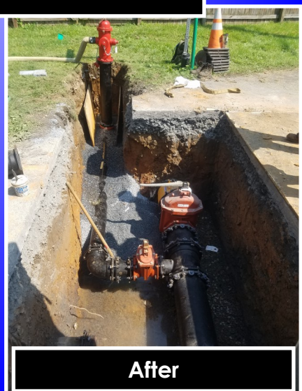
Chestnut Street Valve Replacement & Hydrant Installation
