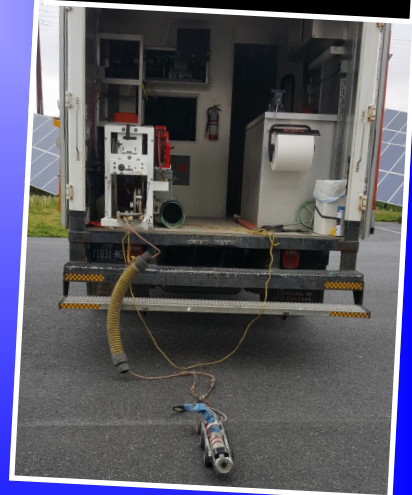
Flushing & Televising of Sewer Mains
