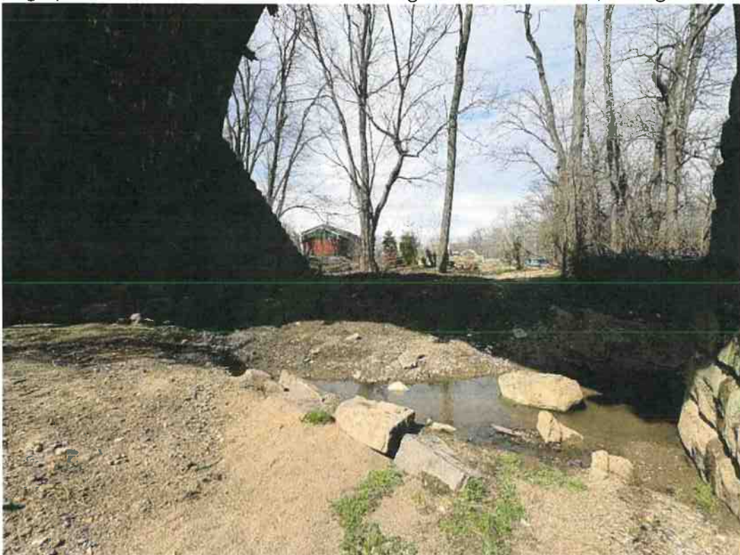
Photograph 6 – View of access road area from under the bridge, facing northeast.
