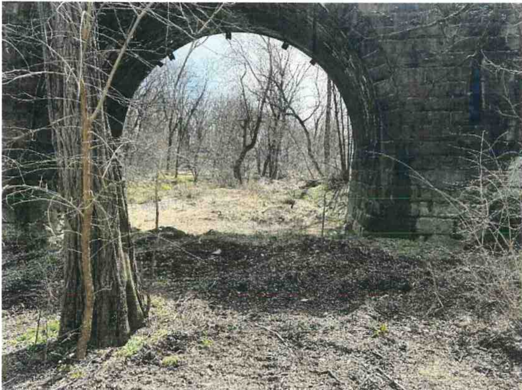
Photograph 4 – View of access road area looking toward the bridge, facing southwest.
