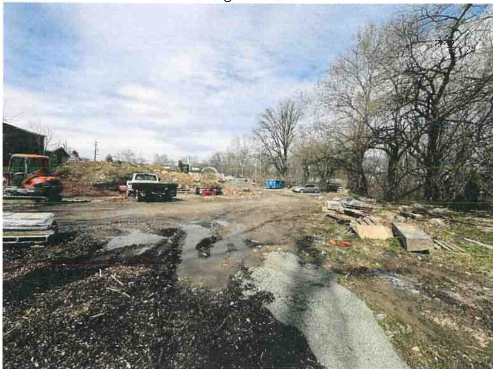
Photograph 2 – View of beginning of access road area toward existing driveway/gravel road, facing northeast.
