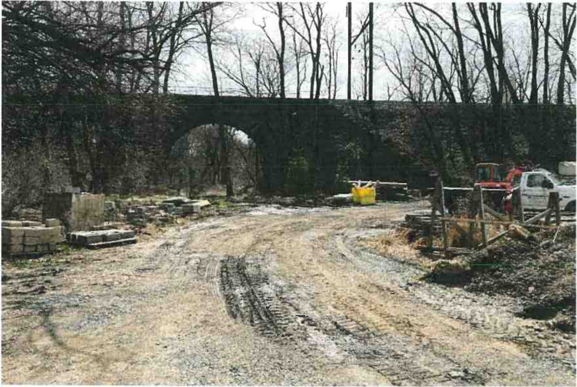
Photograph 1 – View of existing driveway/gravel road toward access road area and bridge, facing southwest.
